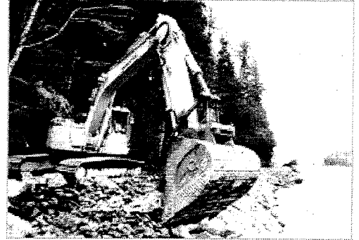
Andrew Pratt, of Quigg Bros. Construction, based in Aberdeen, Wash., uses backhoe Friday, March 7, 2008, to build a rock wall on a bank of the Quinault River where it washed out a portion of North Shore Road in Olympic National Park in Washington state. Even though volunteer crews are making the park the focus of their efforts this year -- joining workers at Mount Rainier and North Cascades national parks in their storm clean-up efforts -- summer visitors will still have to sidestep some storm damage. (AP Photo/Ted S. Warren)
